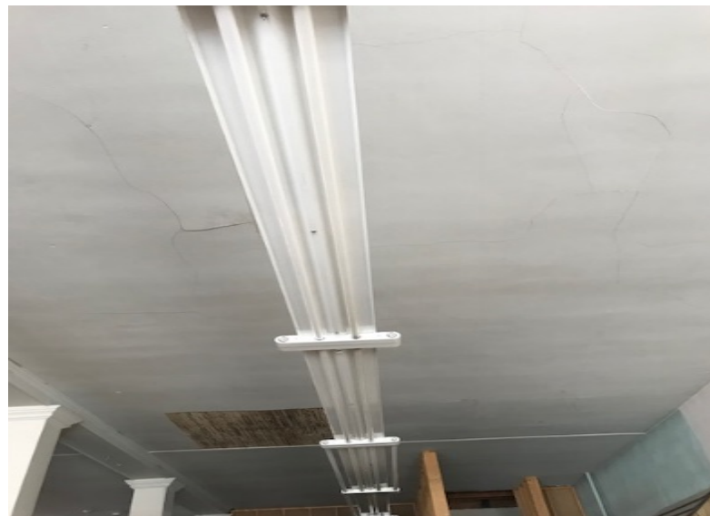
Lighting. Ballasts (PCB containing or otherwise) were not observed but could be present elsewhere among the debris.
