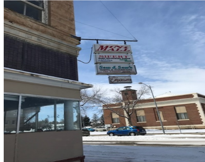
NE corner of subject property looking NW. Note the Mini-Mall sign indicating a prior use.
