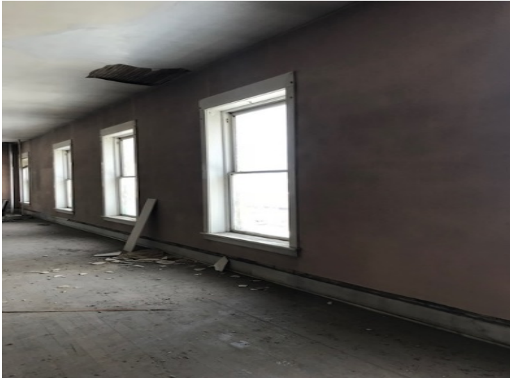
View of upstairs.
