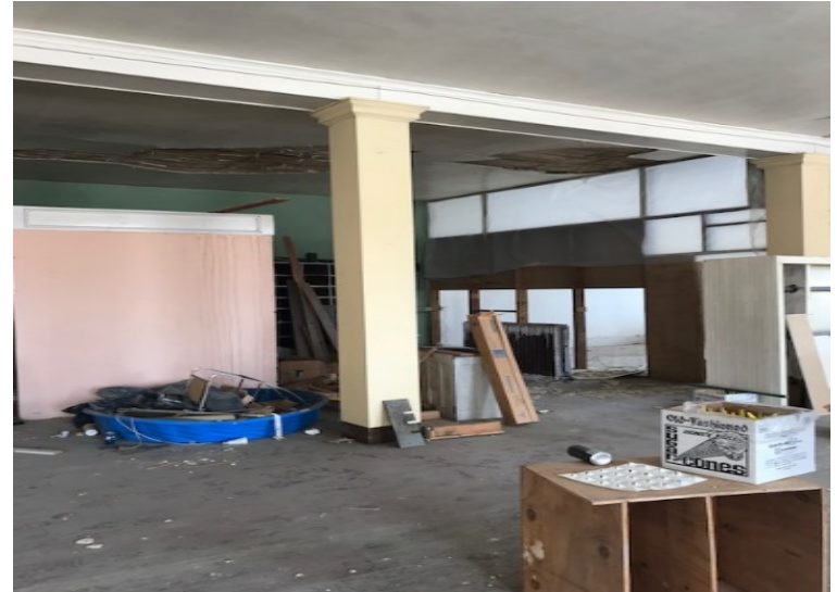
View of upstairs.
