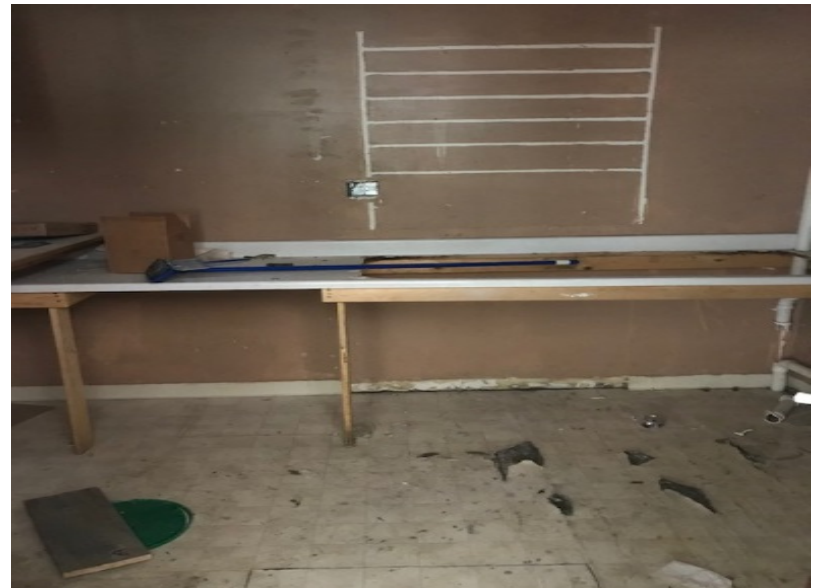
"Kitchen" area off of "Restaurant".
