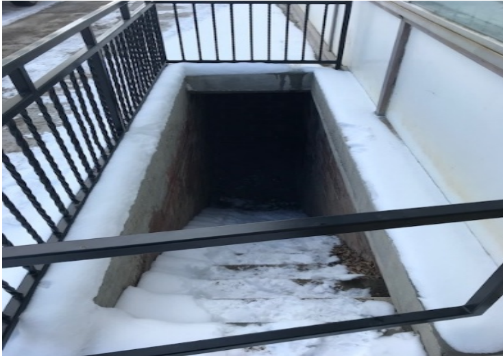
View of subject property access to basement.
