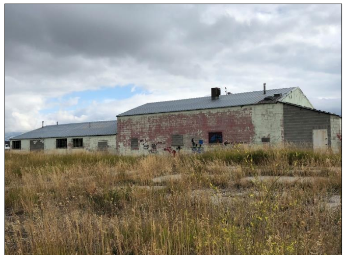
Back View of Nelson Dairy Center Building
