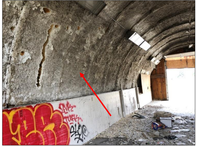
Insulation in Quonset
