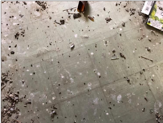
9x9 Floor Tile & Mastic
