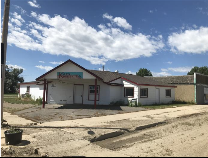
PHOTOGRAPH 1 View of building from street facing SW.
