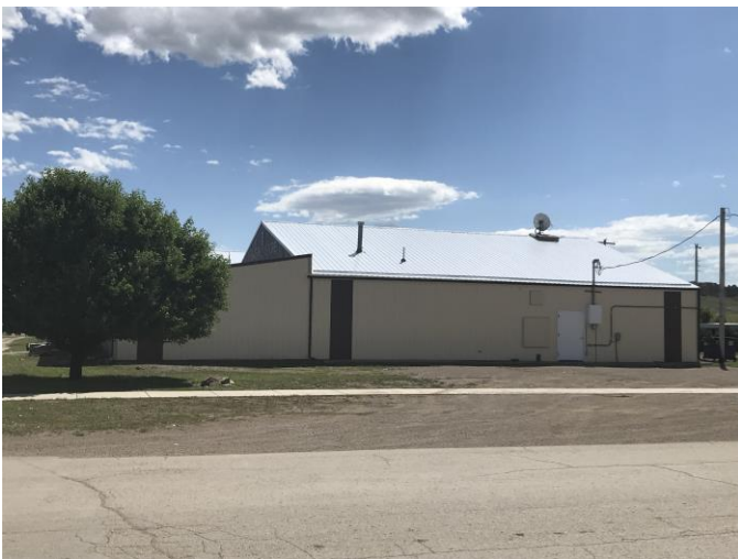
PHOTOGRAPH 5 View across Broadway Ave, facing E.
