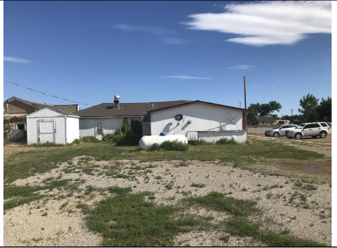
PHOTOGRAPH 2 View from behind building facing N.
