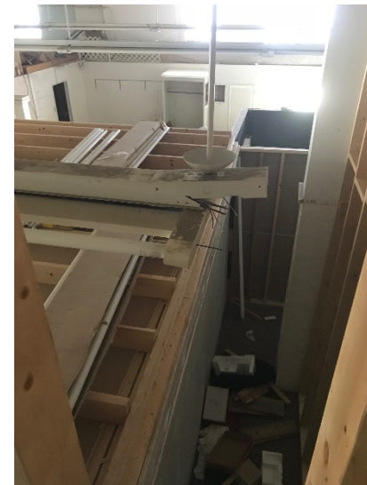
Three rows of similar lighting fixtures on main level.
